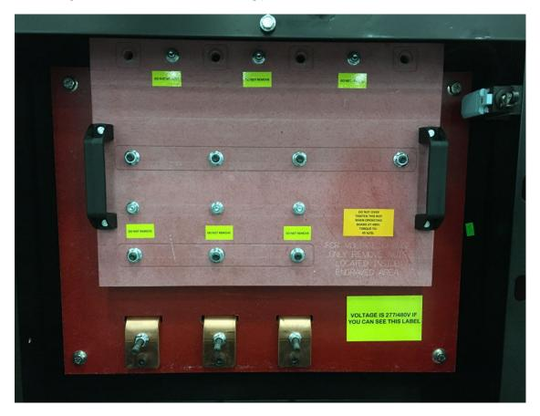
Do not over tighten this nut when operation board at 480V. Torque to 45in/lb Note: Make sure that you see the yellow label with the following message: VOLTAGE IS 277/480V IF YOU CAN SEE THIS LABEL
