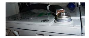
Step 5 Connect the negative (-) Battery cable (blue) to the negative terminal and secure the screw with 10mm insulated wrench.
